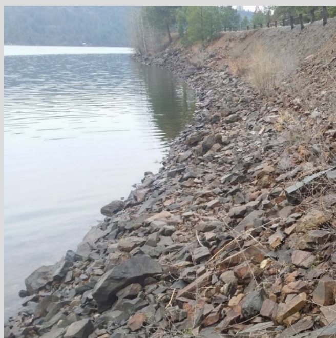
Rip Rap Rock Stabilization
